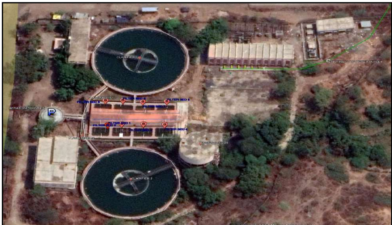
FIGURE 2:8GOOGLE EARTH IMAGE OF PAKHNI WTP
