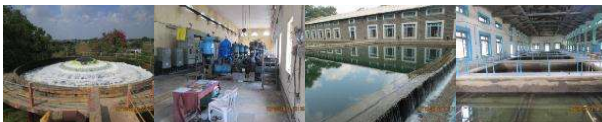
Soregaon Treatment Plant
