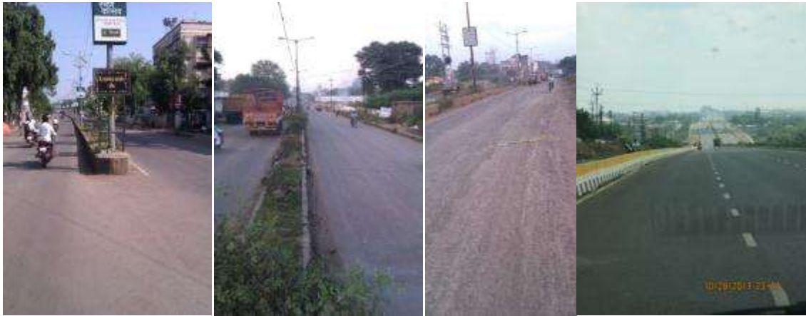
Roads in solapur city
